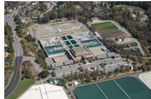
Valley Water Rinconada WTP
